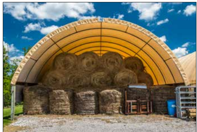
Figure 2-33. Tarp-covered hoop structures provide cost-effective hay storage in Kentucky.
